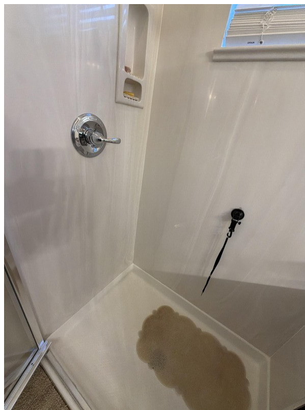
Shower enclosure — clean, good condition
